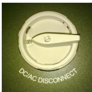
Figure 5.4.9: Turn off DC/AC disconnect switch
