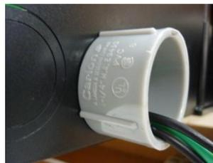
Figure 7.2.4: Insert the AC cables through conduit
